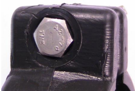
5mm Hex Head bolt in side mount
